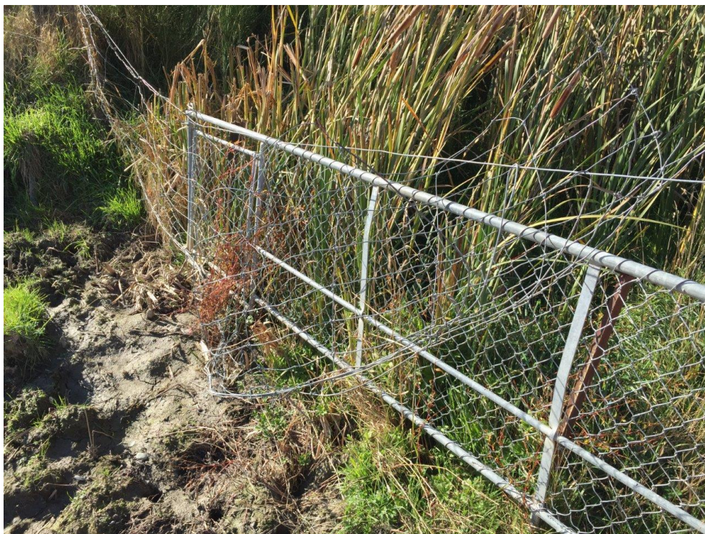
Boundary fence and channel overgrown with Raupo causing silt build up and blockage
